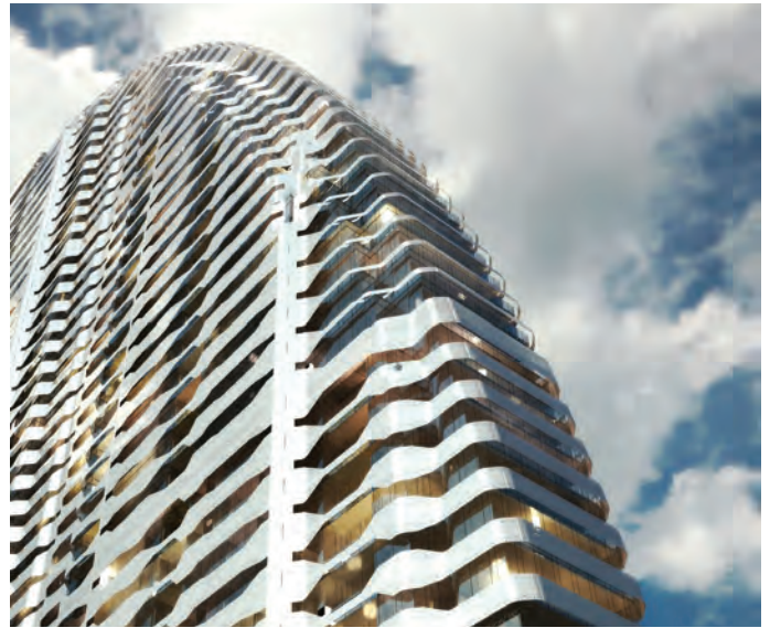
Figure 6. Sunrise: The curved shape presents a receding façade line from street level that does not overwhelm
