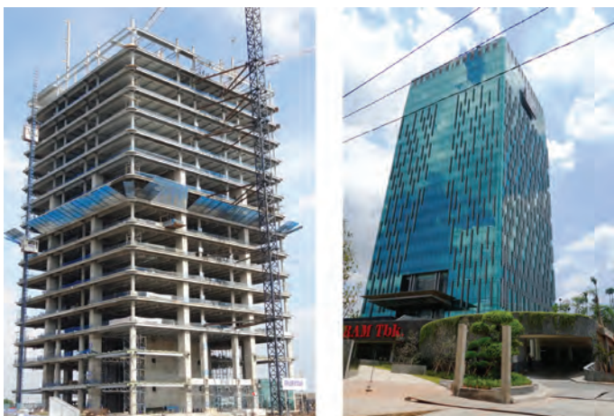
Figure 10. Gudang Garam Office Tower during construction and after completion (Source: Davy Sukamta)
