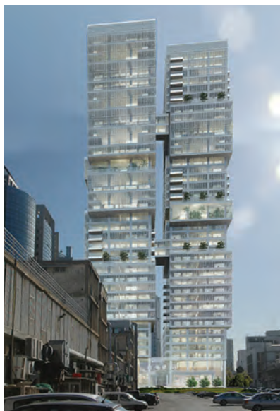
Figure 11. Ha'Arba'a Towers: Study of Multiple Skybridges at Sky Lobby Floors (Source: Moshe Zur Architects & Urbanists)
