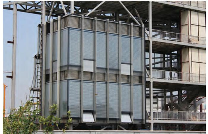
Figure 9. Façade Mock-up Picture. (JAHN)
