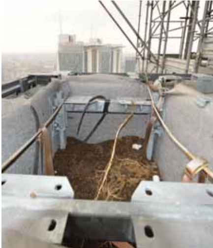
Figure 10. View into a plant container with membrane and protective sheeting.
