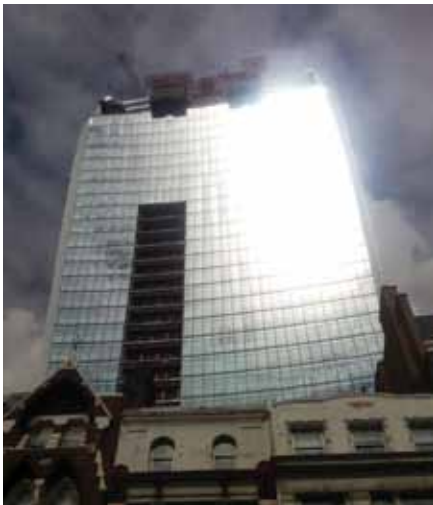
Figure 2. London’s 20 Fenchurch Street’s façade reflects sun rays onto a nearby street. © Simon Price
