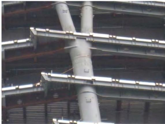
**Photo 2.** Cast steel connection for peripheral tilted column-crossed section.
