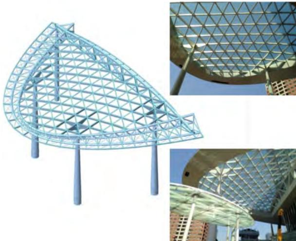
Figure 8. Structural Frame for Large Eave.
