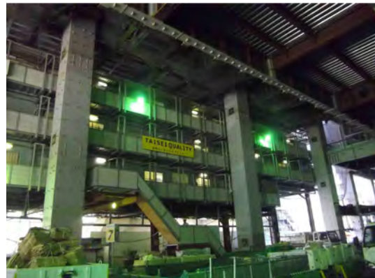
Figure 20. Ultra high strength concrete-filled tubular (CFT) columns.
