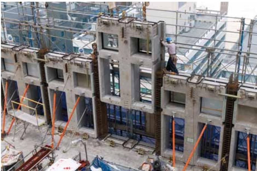
Figure 12. Installation of perimeter precast frames.
