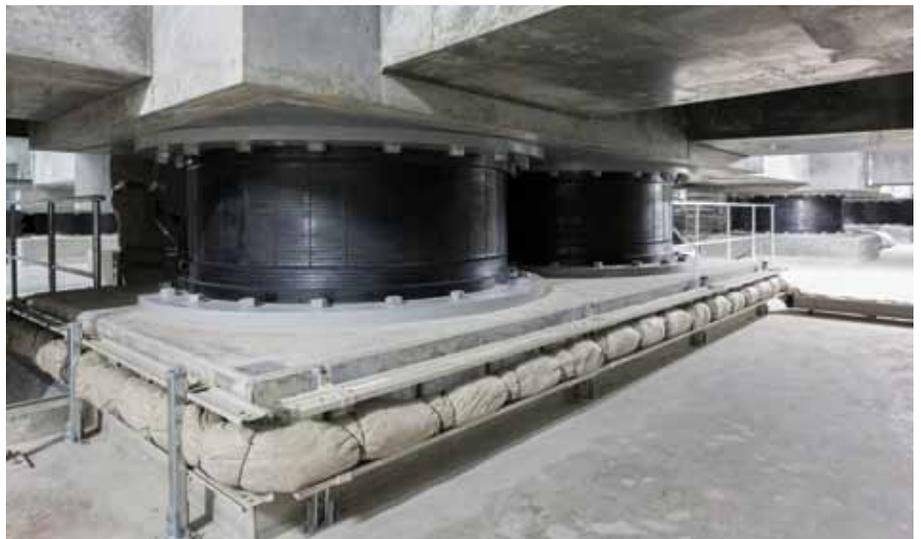
Figure 10. LRBs below core wall.
