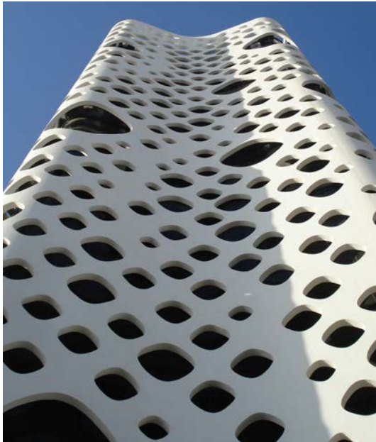
Figure 8. It is nonsensical that we are building towers with all-glass façades, especially in intense solar environments such as the Middle Eastern deserts, then expending more energy installing solar shading to cover up the glass. Tall buildings should concentrate glazing where it is best placed, and introduce more opacity back into the façade, which would also give a greater opportunity for more varied expression, as seen in the 2009 O14 Building in Dubai. Copyright: Reiser and Umemoto.
