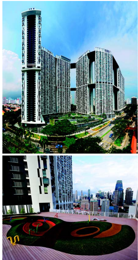
Figure 10. It is nonsensical that we are going ever more vertical in our cities, without introducing the horizontal. Skybridges and Skyplanes give the opportunity for not only linking functions, circulation, services and fire evacuation routes across tall buildings, they can create significant urban habitat in the sky, as evidenced by Singapore's 2009 Pinnacle @ Duxton housing project. Copyright: ARC Studios.
