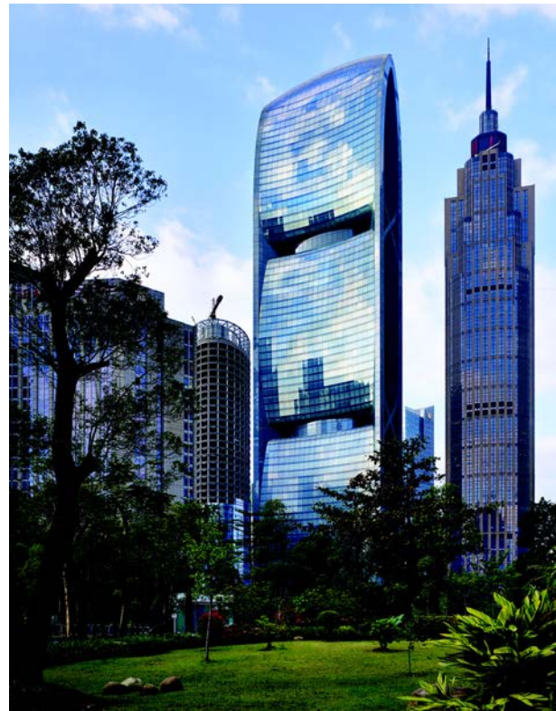
Figure 3. Climatic elements are not only something to be mitigated in tall building design, but can become embraced for positive effect in both the form and operation of tall buildings; natural energy capture, natural ventilation, rain-water capture etc. The strategies and systems to enable this can influence the design and expression of the building. Pearl River Tower, Guangzhou (2013) demonstrates several of these ideas. Copyright: SOM.
