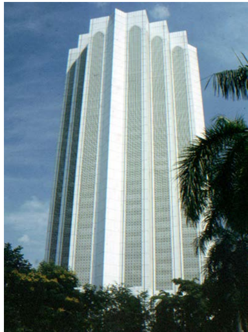
Figure 4. Tall Buildings can reflect the local culture in a literal way - as demonstrated here with the 1984 Dayabumi Complex in Kuala Lumpur with its façade a modern interpretation of the Islamic jali screen - or in a more direct way, by incorporating specific activities and ways of life into the program of the building. Copyright: Antony Wood.
