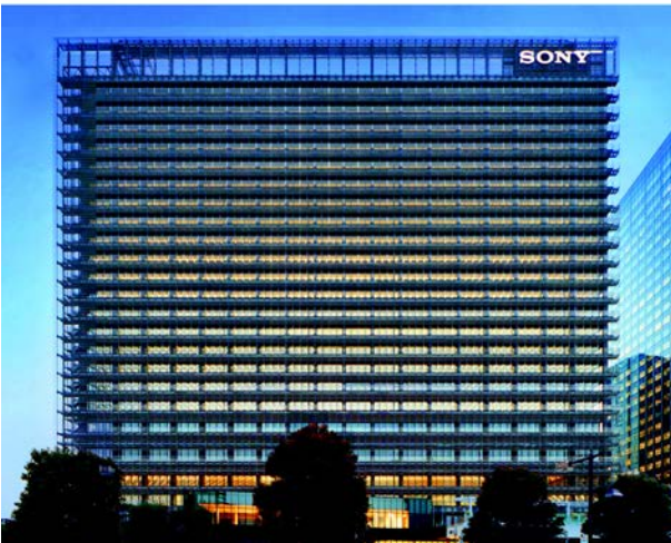
Figure 6. Every expenditure of carbon through the embodied energy in materials and systems needs to be justified by overlaying more usage on those systems. In the 2011 NBK Osaki Building in Tokyo, the “Bioskin” solar shading shields internal spaces from solar gain and, through the system containing recycled rainwater, simultaneously reduces the external urban heat island effect through evaporation. Copyright: Nikken Sekkei.
