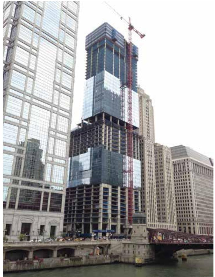
Figure 13. Curtain wall installation in two, later three stacks with three separate crews (Source: Handel Architects)
