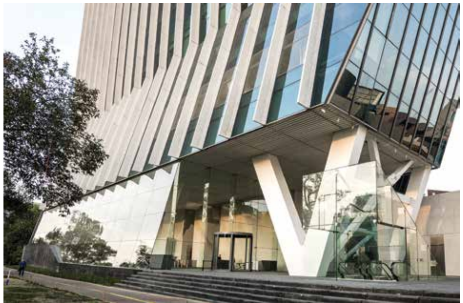
Figure 5. The V brace at 24 Pedregal (Source: CAMILA COSSIO)
