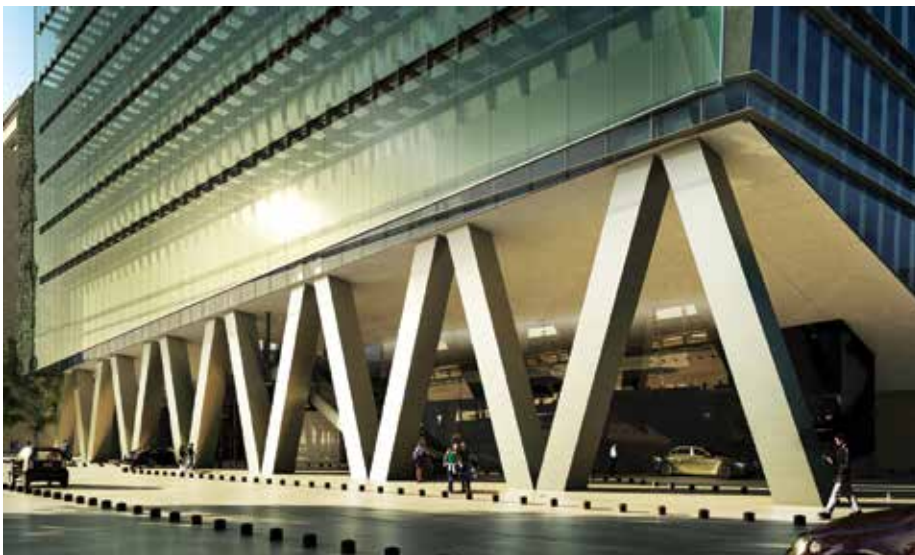
Figure 3. The ground floor of Reforma 509 has no internal columns allowing passenger drop-off and facilitating mechanized parking below ground. (Source: Arup)
