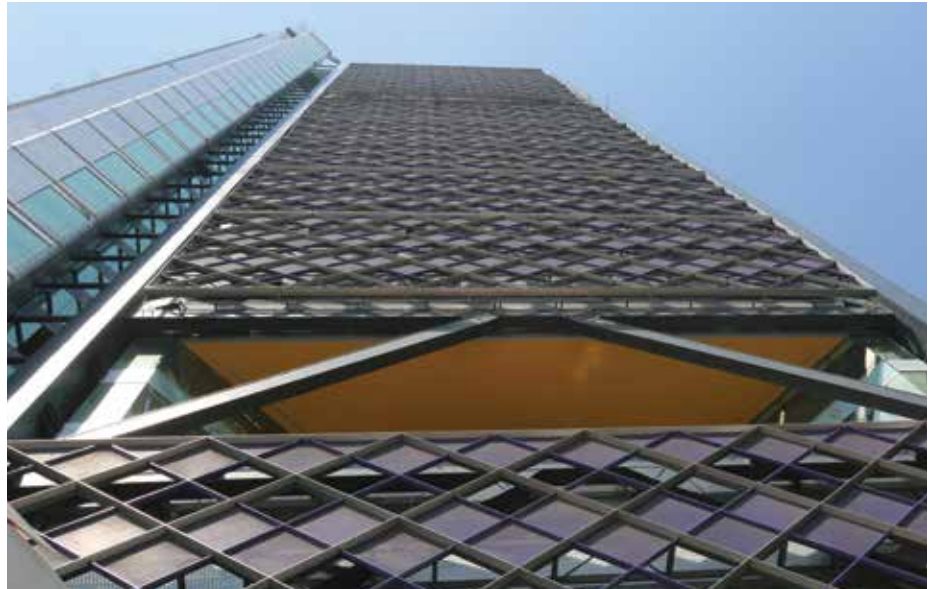
Figure 4. Torre BBVA Bancomer uses an Eccentrically Braced Mega frame to provide lateral stability and flexibility of floor planning. (Source: Arup)
