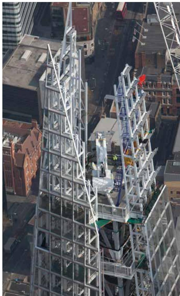
Figure 8. Placing last piece of steel on the spire (Source: Sellar Property Group)
