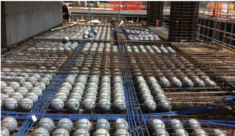
Figure 9. The low weight post-tensioned slabs (Source: ECSD)
