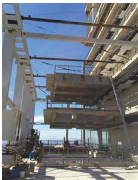
Figure 10. The post-tensioned jump-deck slabs floors (Source: ECSD)
