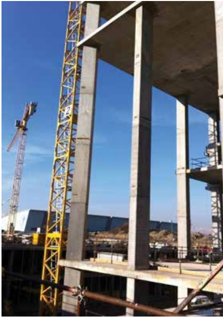
Figure 7. Slender columns with composite section (Source: ECSD)
