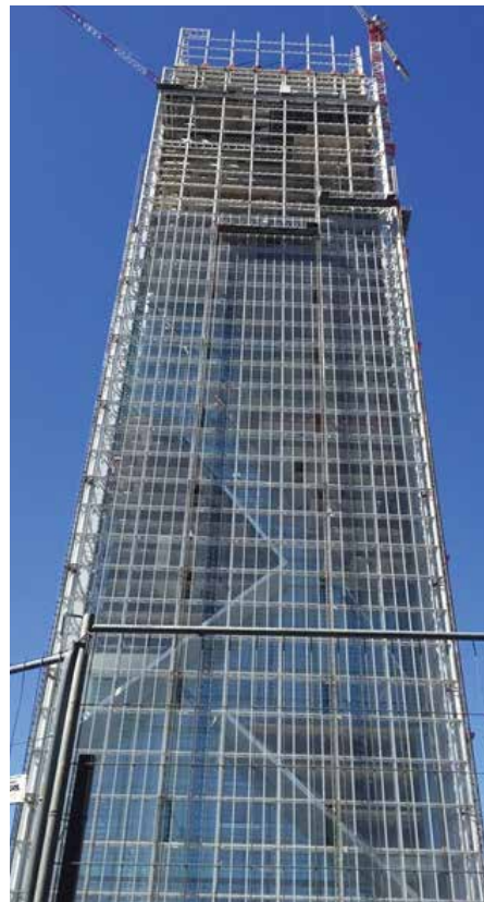
Figure 4. External view of the East Facade (Source: ECSD)
