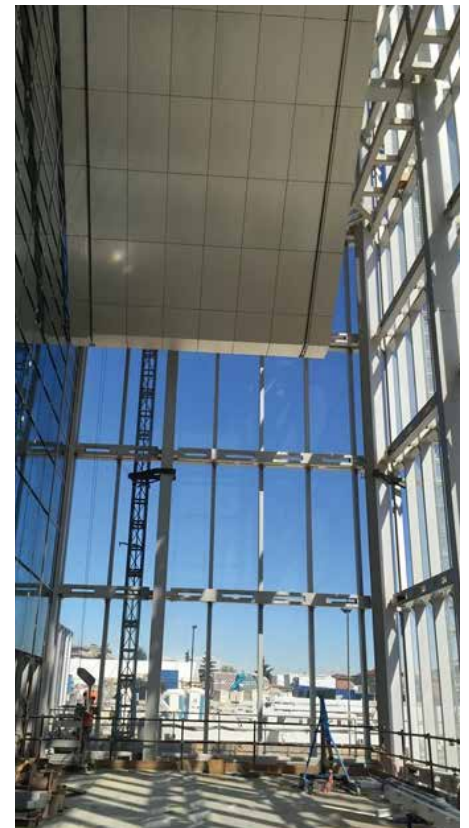
Figure 5. The interior view of the East Facade (Source: ECSD)
