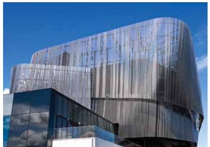
Figure 7. Stockholm Congress Centre used duplex 2205 sunscreens for better corrosion performance. © Outokumpu
