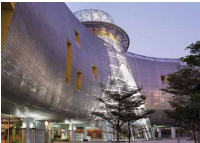
Figure 6. Guangzhou, China's Second Children's Activity Center was wrapped in stainless steel mesh to reduce energy requirements and create a seamless sculptural shape. © Steffian Bradley Architects
