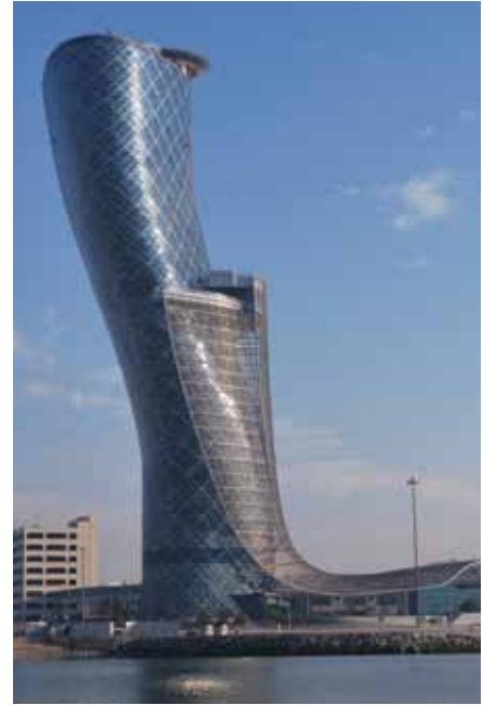
Figure 4. Woven stainless steel sweeps down from the 19 th floor of Abu Dhabi's Capital Gate Tower, reducing energy requirements. © Jeff Schofield
