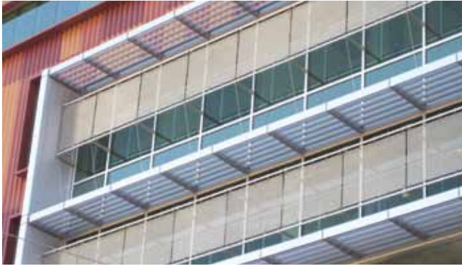
Figure 5. Type 316 sunscreens shield windows on the Cronkite building at Arizona State University (ASU). © GKD
