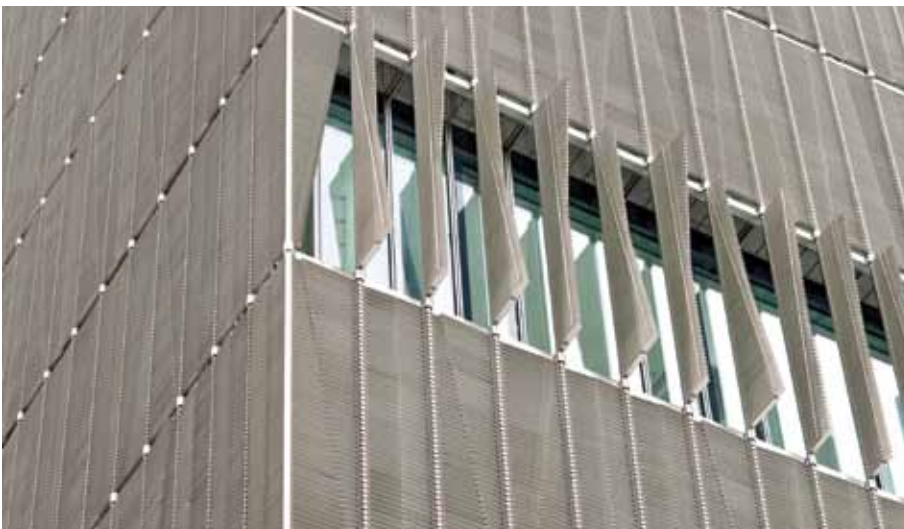
Figure 1. Type 316 stainless steel exterior sunscreens in varying styles were used on the ThyssenKrupp corporate campus to actively adjust to seasonal and weather conditions to reduce energy requirements. © ThyssenKrupp AG
