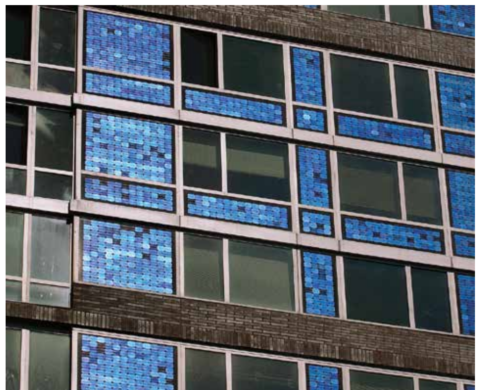
Figure 4. The Solaire, Pelli Clark Pelli, View of vertical photovoltaics (Source: FXFOWLE)
