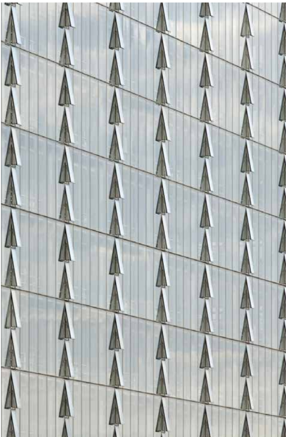
Figure 10. Manitoba Hydro Place, KPMB Architects. View of Operable Windows. (Source: Tom Arban)
