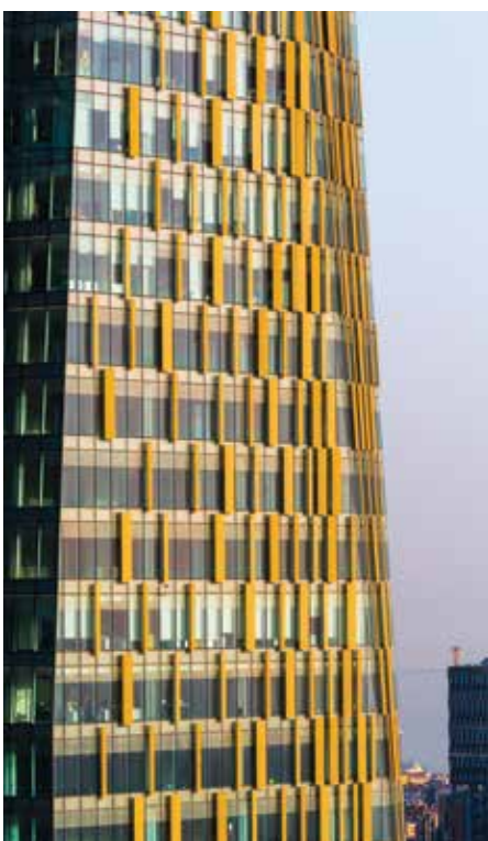
Figure 3. Allianz Tower, FXFOWLE Architects. View of exterior shading (Source: FXFOWLE, credit: David Sundberg/Esto)
