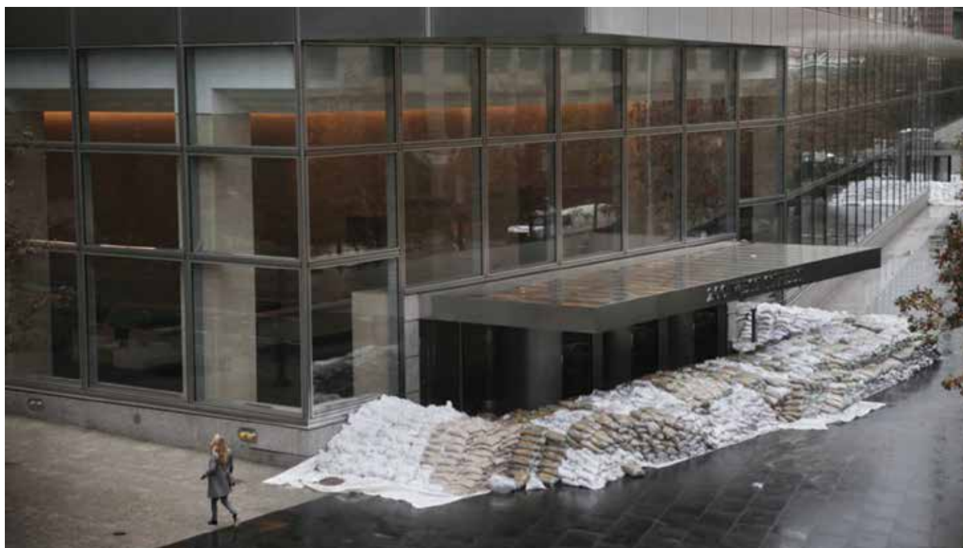
Figure 12. Sandbagged entry of Goldman Sachs Headquarters prior to Superstorm Sandy (Source: Victor J. Blue/Bloomberg)
