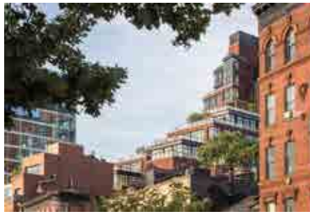
Figure 5. 150 Charles Street, construction view, June 2015 (Source: COOKFOX Architects)
