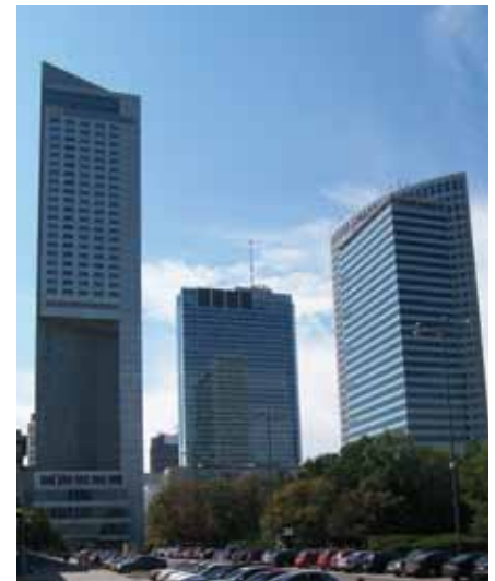
Figure 5. Three new skyscrapers built in the Western City Center after 1989 – (from left): InterContinental Hotel, Rondo 1, and Warsaw Financial Center. © Wojciech Olenski
