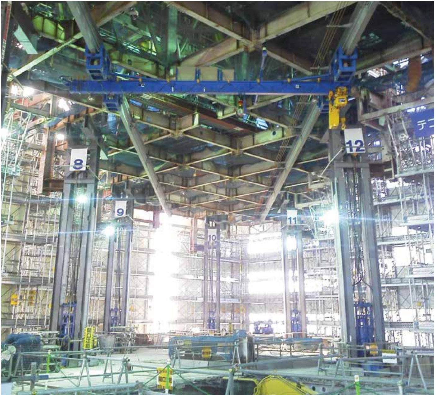
Figure 15. The utilization of the existing roof structure (Source: Taisei Corporation)
