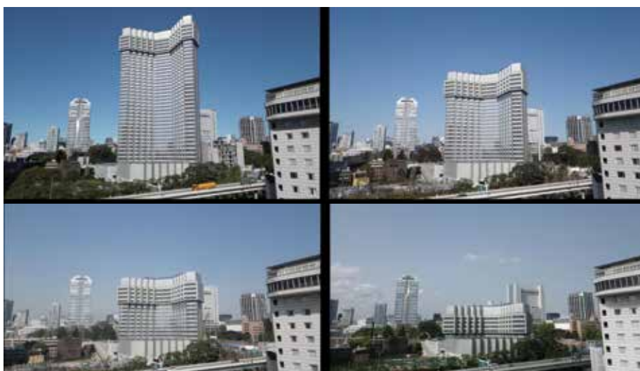
Figure 14. Work proceeding situation (Source: Taisei Corporation)
