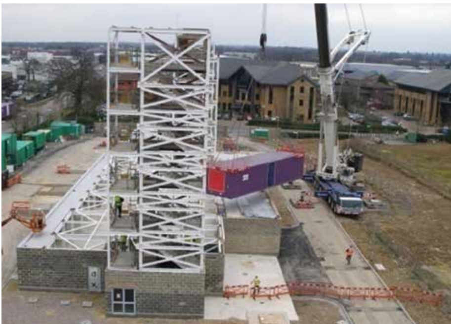
Figure 6B. Modular stability systems
