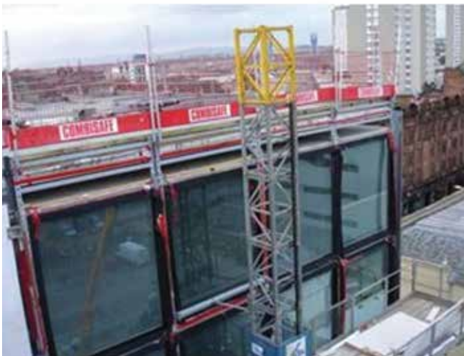
Figure 8. CitizenM Glasgow – mast climbers installing cladding (Source: Ramboll Group)
