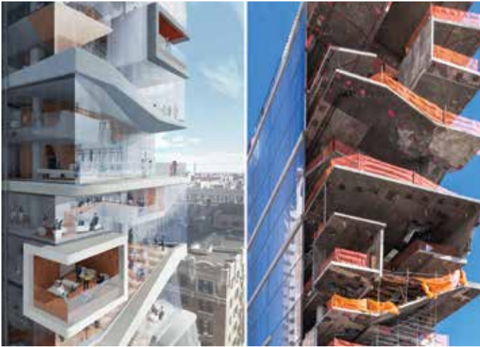
Figure 10. Form and function of the Cascade: the architectural design manifested through the structural interconnection between floors (Source: Diller Scofidio + Renfro left /Fadi Asmar right)
