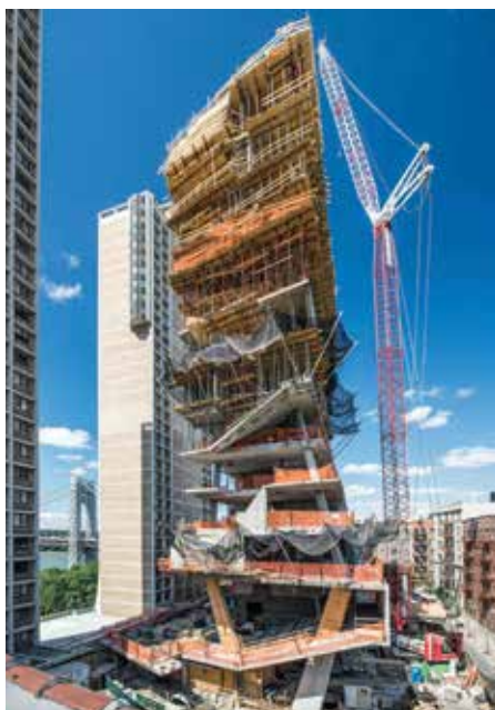
Figure 6. Cascade reshoring during construction (Source: Matthew Melrose)
