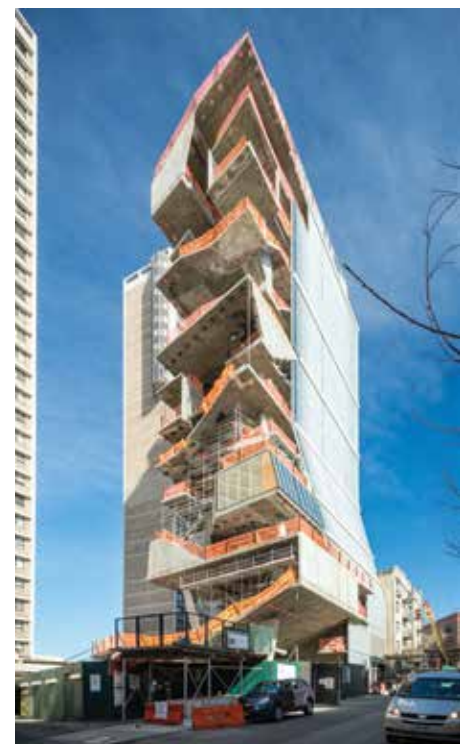
Figure 4. South elevation showing cantilevered slabs with varying floor-to-floor slab edge positions (Source: Matthew Melrose)
