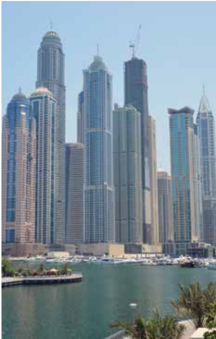
Although the density of Dubai is often criticized, there are distinct benefits to the close spacing of the narrow, square plan towers that have evolved. In Marina Bay these provide much needed shade in an environment that does not naturally support vegetation. (Source: Terri Meyer Boake)
