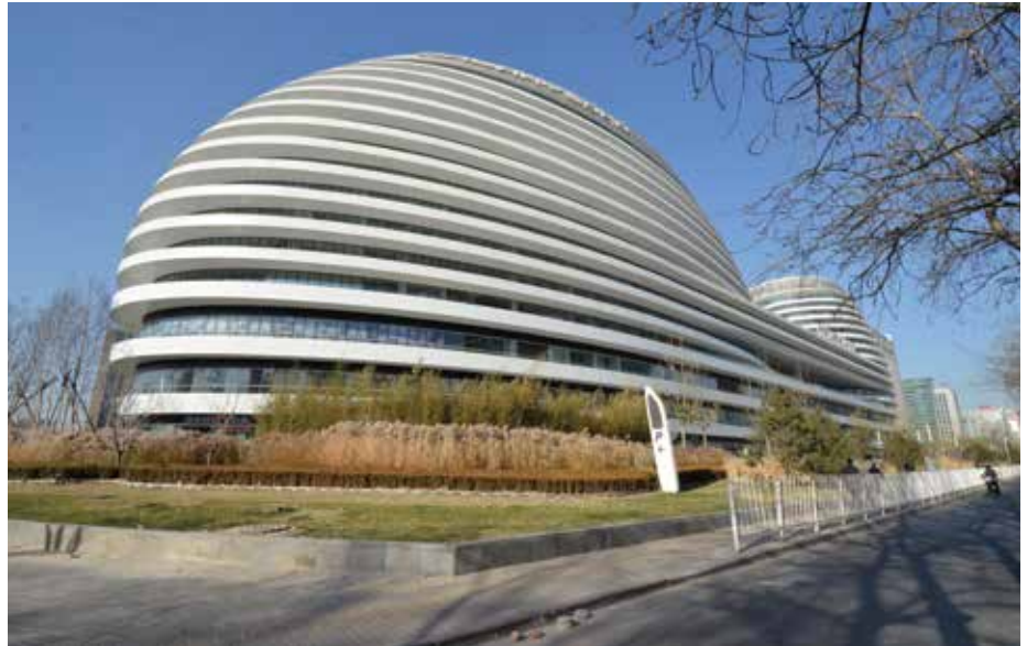
Galaxy SOHO in Beijing, China fails to engage or activate the urban environment due to its inward looking retail program and barrier like landscaped setback from the sidewalk. (Source: Terri Meyer Boake)
