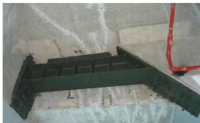
Figure 15. Cracked perimeter girder reinforced with steel member (Source: Daewoo E&C)
