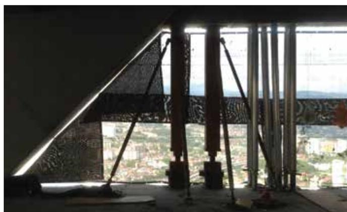
Figure 14. Temporary installation of support under perimeter girder (Source: Daewoo E&C)
