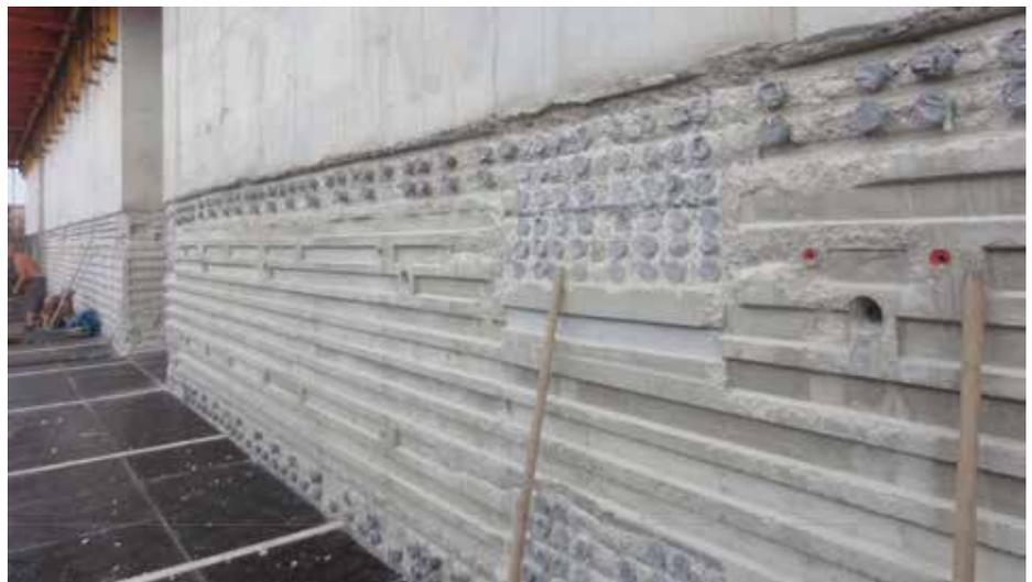
Figure 16. 3D-Rebar Design: Core Walls and Connection to Outrigger Slab (Source: Bollinger + Grohmann)
