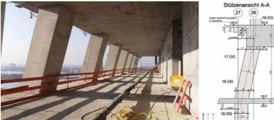
Figure 8. Inclined Columns at the Folded Façade (Source: Bollinger + Grohmann)
