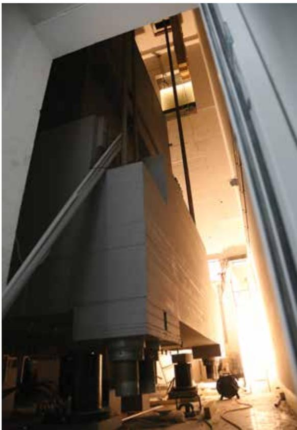
Figure 19. Tuned Mass Damper of the DCT 1 (Source: Bollinger + Grohmann)
