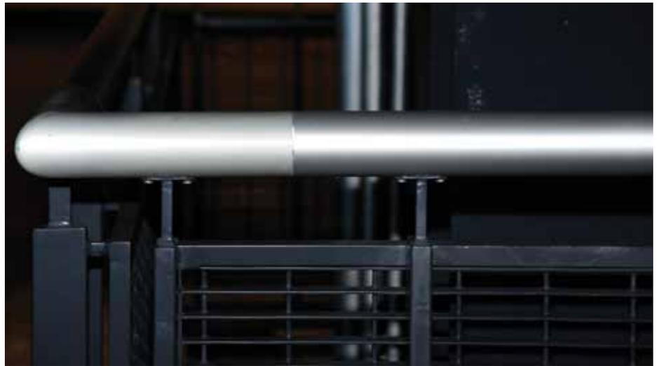
Figure 11. Naturally occurring color variations in newly installed anodized aluminum (Source: AkzoNobel)
