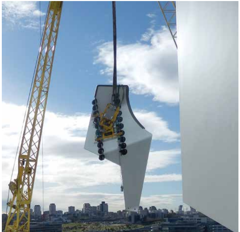
Figure 14. Installation of the fins on-site (Source: ENvolventes ARquitectonicas - ENAR)
