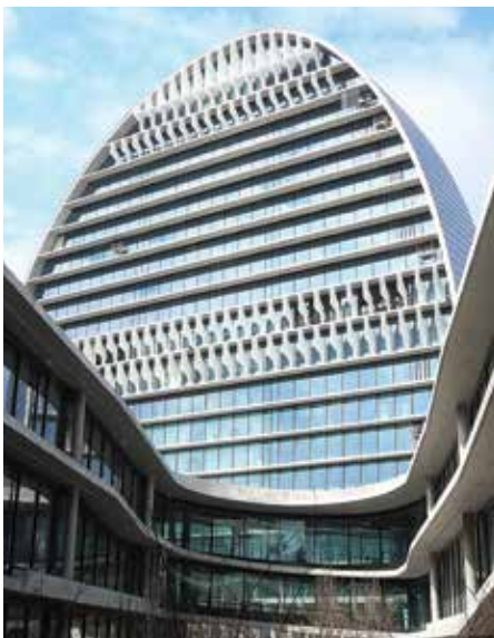
Figure 1. Interior view of the building complex (Source: ENvolventes ARquitectonicas - ENAR)
