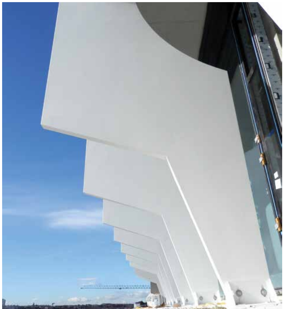
Figure 15. Installation of the fins on-site (Source: ENvolventes ARquitectonicas - ENAR)
