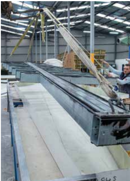
Figure 11. Placing the interior structure of the fins (Source: ENvolventes ARquitectonicas - ENAR)
