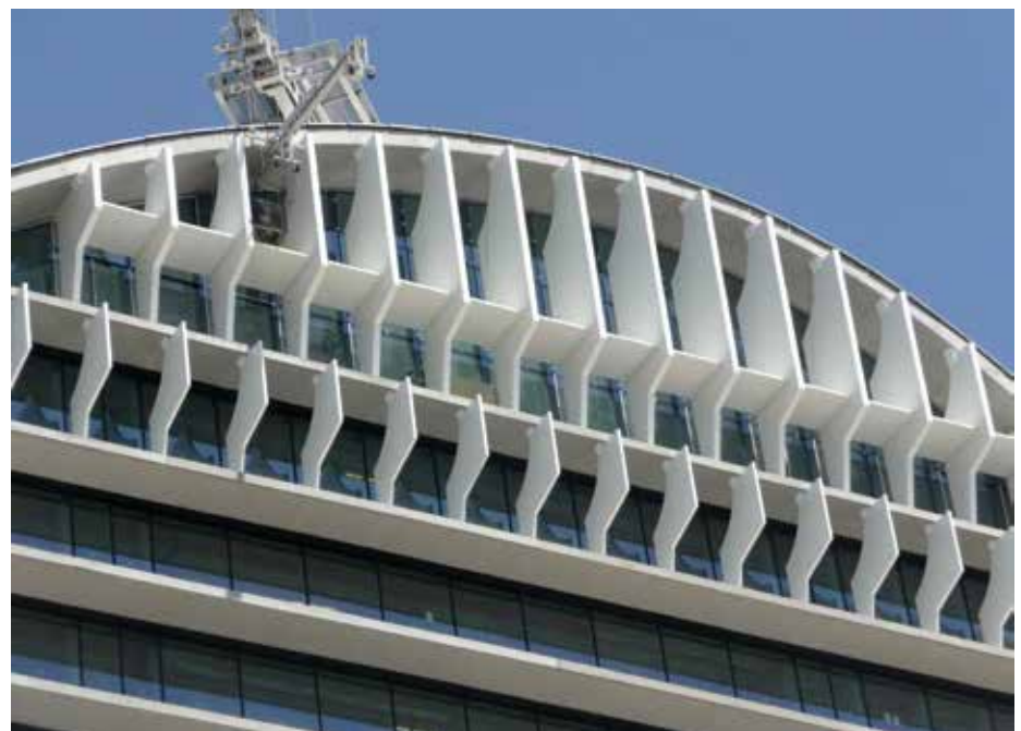
Figure 2. View of the shading elements on the top of the building (Source: ENvolventes ARquitectonicas - ENAR)
