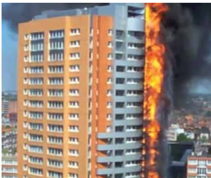
Figures 4, and 5. Combustible Exterior Wall Fires (Source: National Fire Protection Association)
