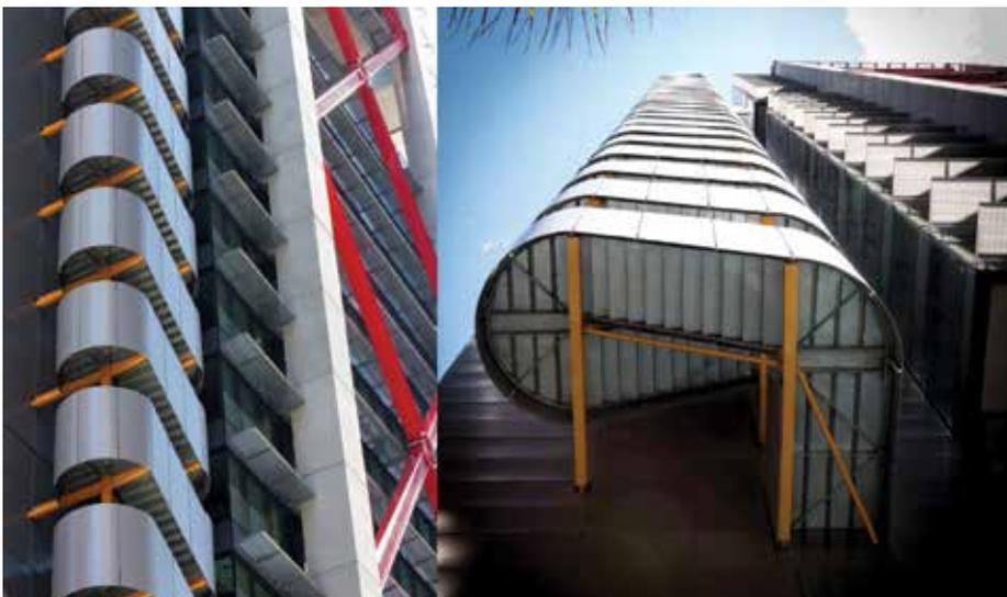
Figure 11. Exterior steel fire stairs (Source: Brett Boardman)
