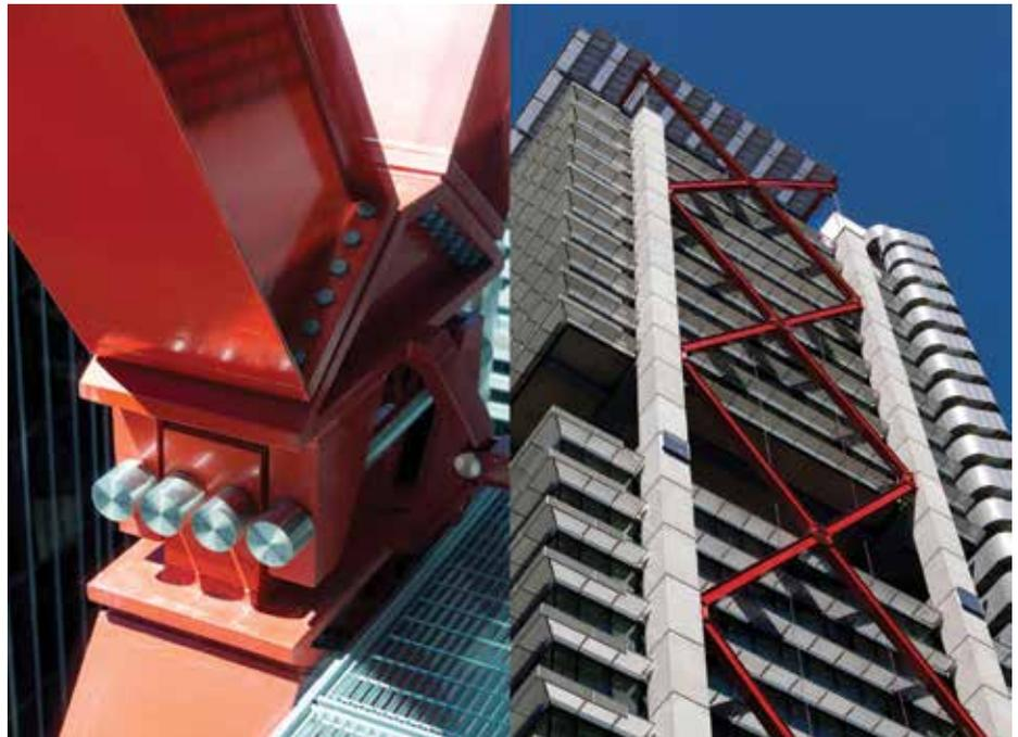
Figure 7. Pinned link node (Source: Brett Boardman)
