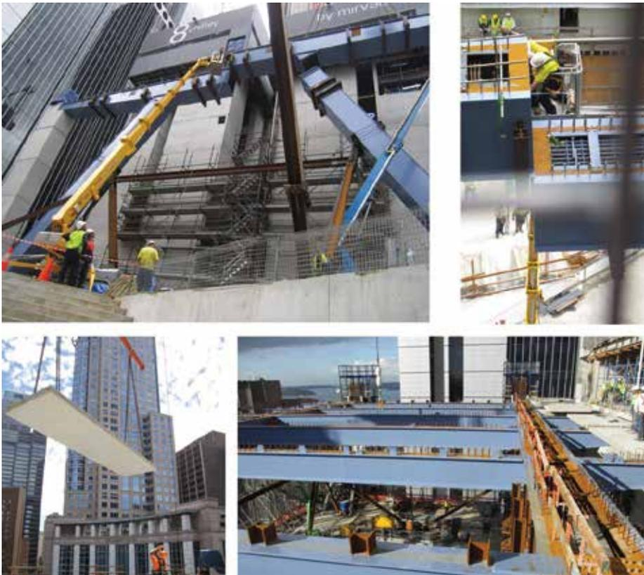
Figure 10. Composite megaframe assembly (Source: Arup)
