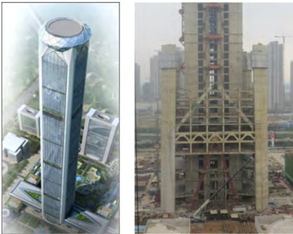
Figure 8. BRB in Tianjin Goldin 117.
