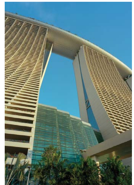
Figure 7. View looking up at the "Belly"
