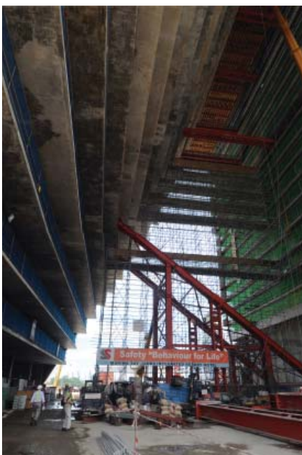
Figure 10. Temporary steel struts for the sloping towers
