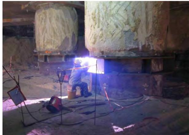
**Figure 21.** Welding of bracket for beam/slab reinforcement connection.
