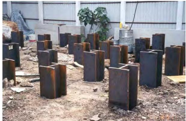
**Figure 5.** Snapshot of a site using percussive steel H-pile foundation.
