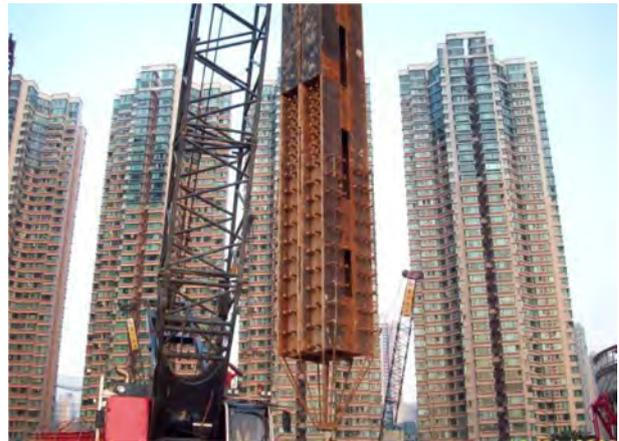
**Figure 13.** Stanchion installation into Bored Pile.
