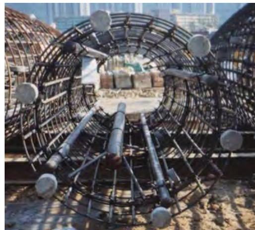
**Figure 3.** Reservation pipe within bored piles.
