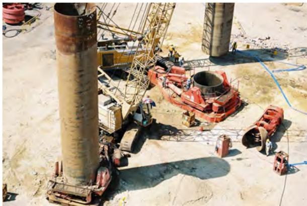
**Figure 1.** Overview of constructing large diameter bored pile foundations.
