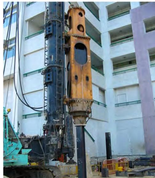
**Figure 6.** Pile pitching using hydraulic hammer.
