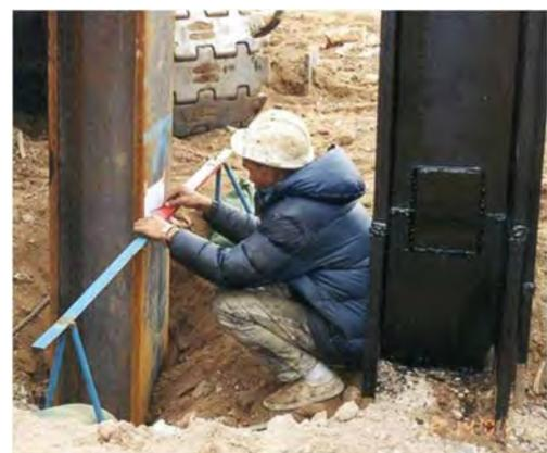
**Figure 7.** Final setting of pile.
