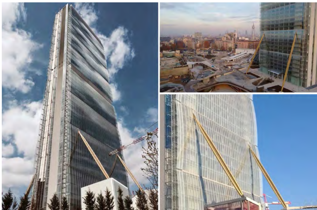
Figure 3. Outer bracing system.
