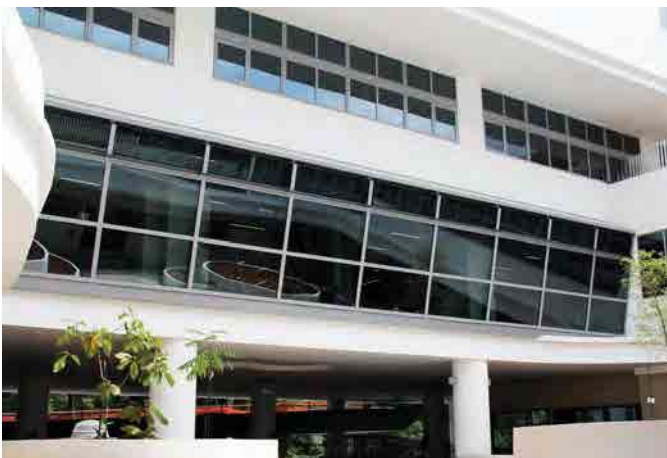
Figure 3. Photo of constructed 3for2 pilot façade at UWCSEA in Singapore, 2015.
