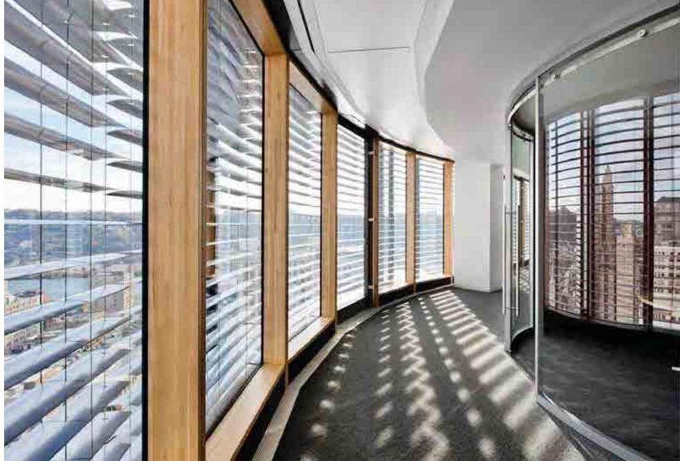
Figure 14. Wooden mullions provide embodied energy savings and a unique, enhanced aesthetic.
