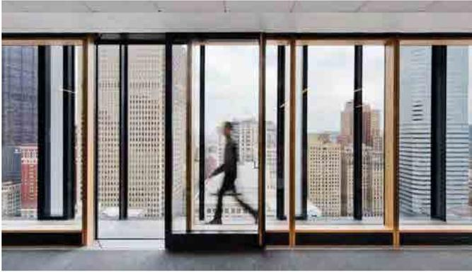
Figure 8. Operable doors in the double façade. © Connie Zhou Photography
