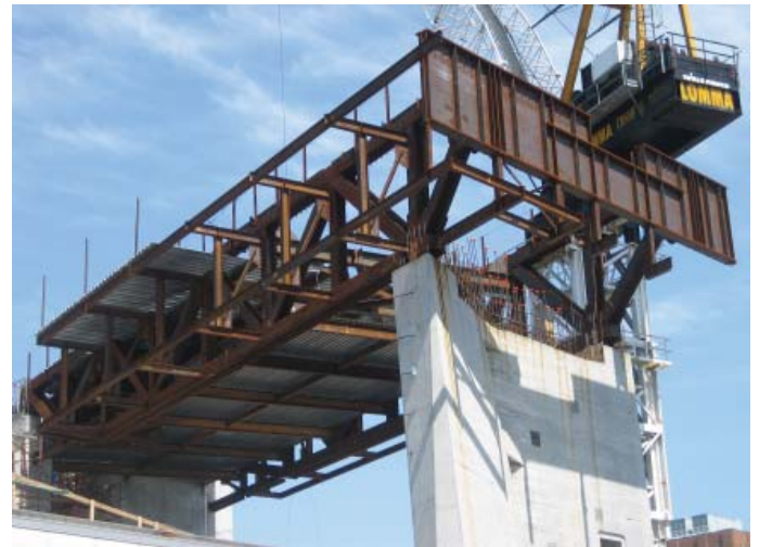
Figure 7. 114' Truss Spanning the Highline © Craig Tracy / DeSimone
