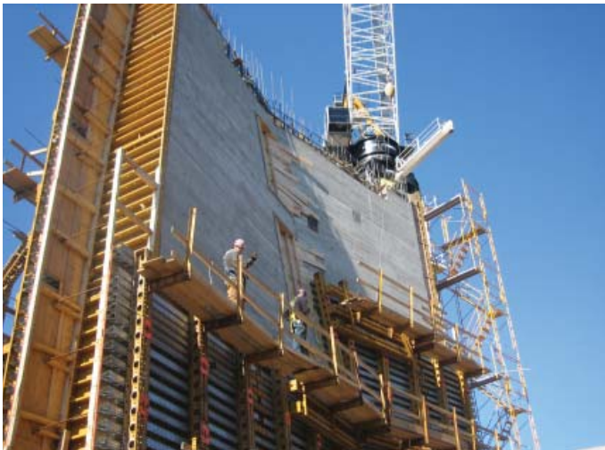
Figure 6. Construction of 60' Tall Sloping Wall © Dominic Buenaventura / DeSimone
