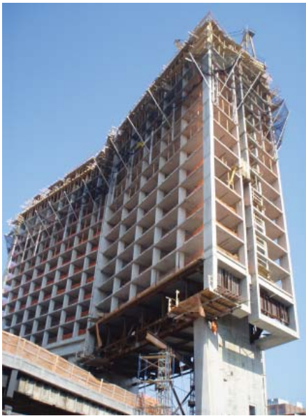
Figure 4. Tower Erection above the Highline © Dominic Buenaventura / DeSimone
