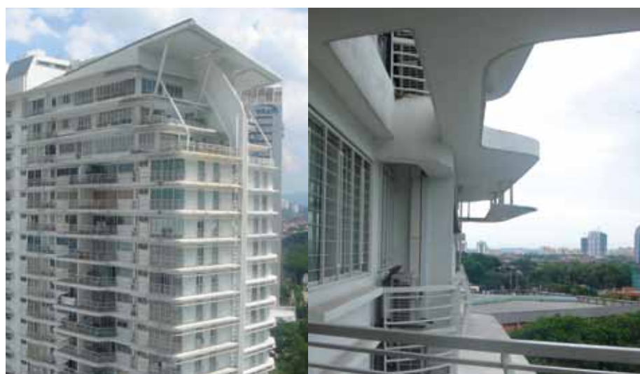
Figure 6. TTDI tower, north-south orientation, white façades and shading devices to reflect incident solar radiation © T.R Hamzah and Yeang
