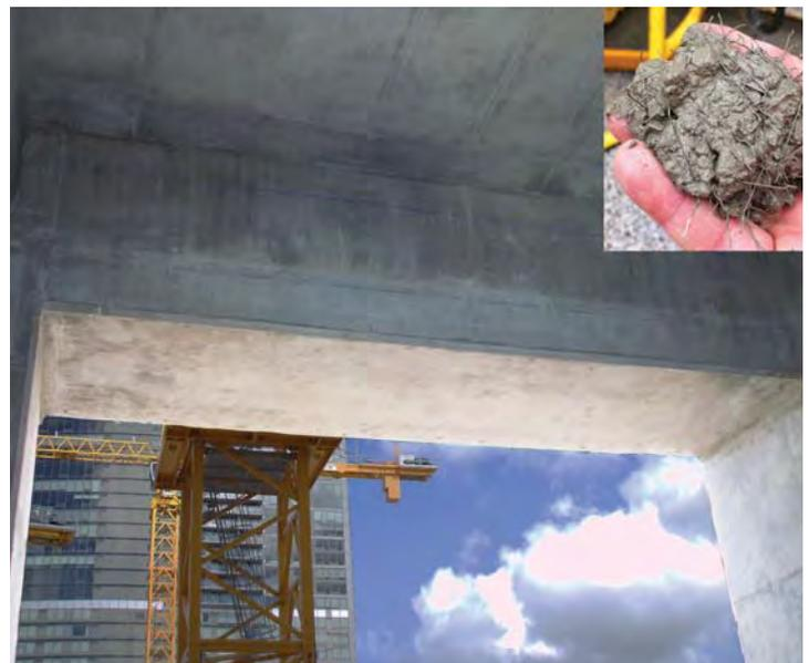
Figure 4. Steel-fiber reinforced concrete (SFRC) coupling beams.
