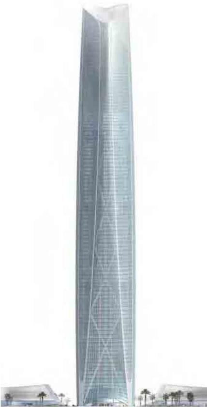
Figure 3. Haikou Tower rendering showing megacolumns with diagonal bracings.
