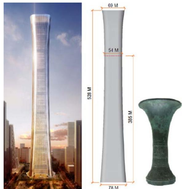
Figure 1. Rendering elevation view and the size of “Zun” (© Kohn Pedersen Fox Associates).
