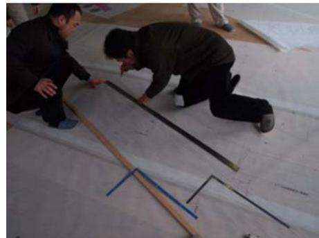
Photo 9. Entering structural steelwork onto full size drawing.
