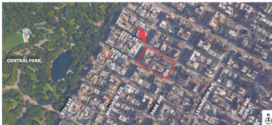
Figure 4. A typical Manhattan city-block combines variety within the order of the grid. Buildings within the block are situated to allow for light and air while responding to the hierarchy of streets; lower buildings are situated on narrower east-west streets, while taller buildings mark the ends of the blocks along wider avenues. The system is occasionally punctuated by a taller building, here the tower of the Carlyle Hotel, which serves as a visual marker for the surrounding neighborhood. (Source: Google Earth, RAMSA)
