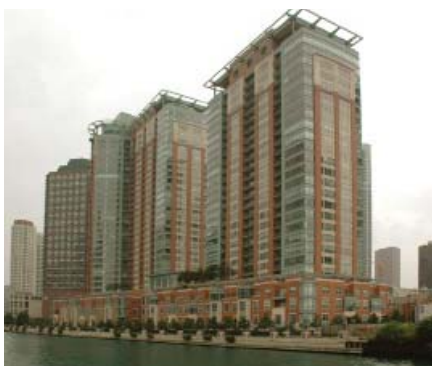
Figure 9. Cityfront Place, Chicago. Slabs are set back and lined with townhouses creating a pedestrian scale base – also known as the Vancouver model © Moule & Polyzoides
