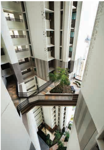
Figure 8. Skyville @ Dawson, Singapore was designed as a "breezeway tower." © Patrick Bingham-Hall
