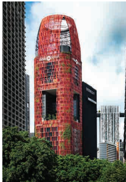
Figure 9. The Oasia Tower, Singapore has a "breezeway atrium" at the top, and its exoskeleton offers an alternative to full glazing. © Patrick Bingham-Hall
