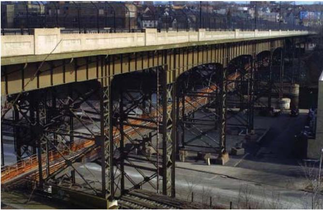
Figure 4. Holton Viaduct, Milwaukee with the Marsupial Bridge suspended below © Jim Brozek
