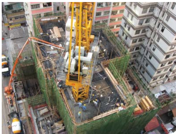
Figure 2. York Place under construction and completed
