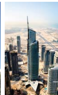
2. Almas Tower Dubai, UAE 363m / 1191ft
