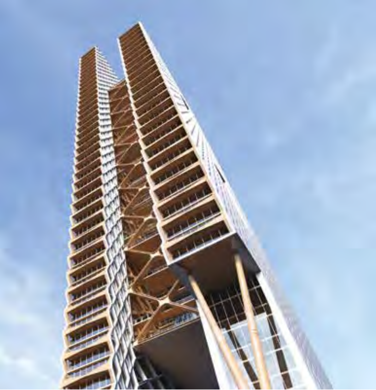
Figure 4, Atrium cross-bracing is key to both the stability and the architectural expression of the design. © Perkins+Will
