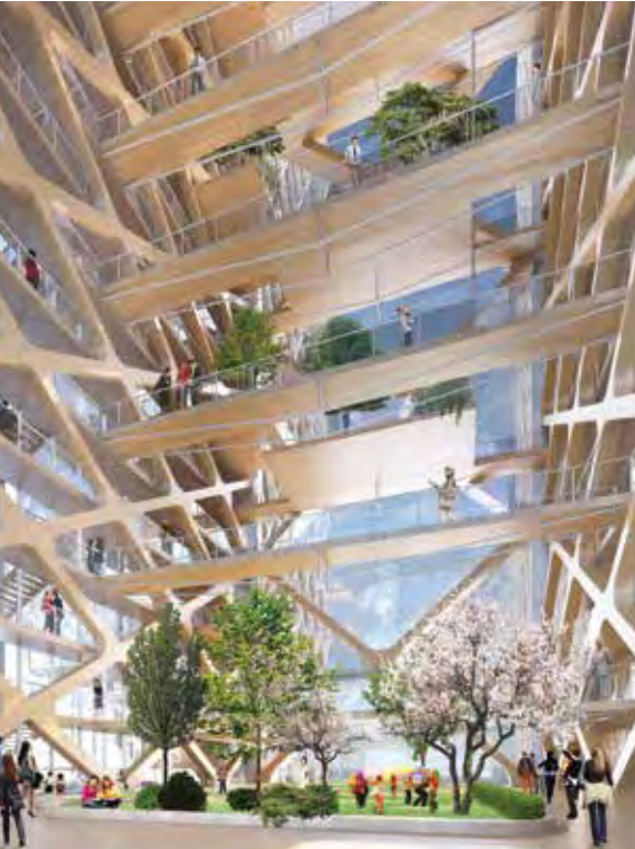
Figure 9. The braced area between the two towers required for stiffness is activated as an atrium amenity space. Exposed wood surfaces emphasize mass timber's expressive potential. © Perkins+Will
