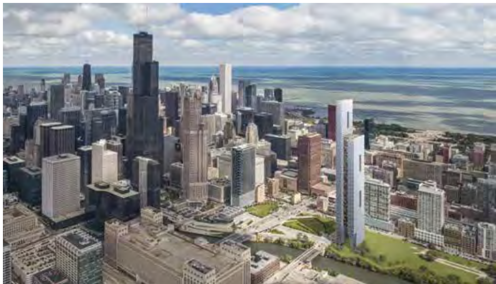
Figure 2. The proposed tower in context of its site at the southwest edge of the Chicago Loop CBD. © Perkins+Will
