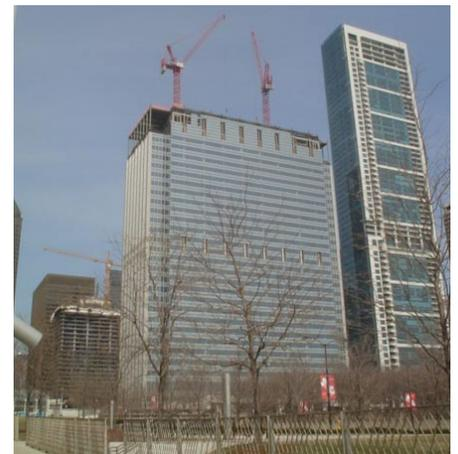
Figure 3. Blue Cross Blue Shield at start of vertical expansion
