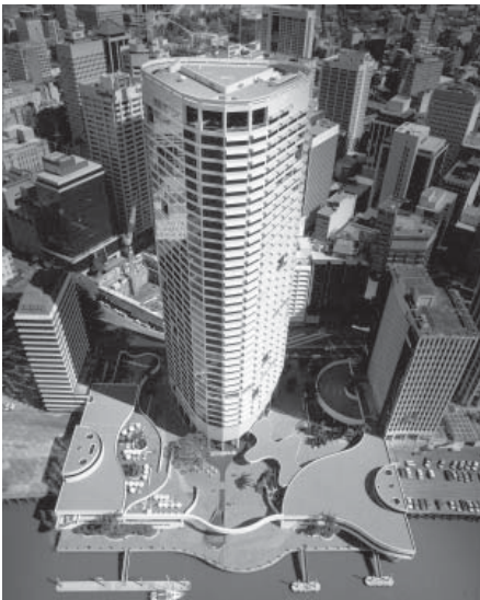
Figure 5. Riverside Development, Brisbane, 1986, by Harry Seidler. Aerial photo. © Harry Seidler Associates
