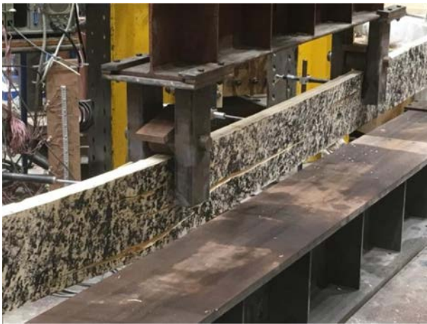
Figure 12. Failure mode of a Glulam undamaged control beam, whose failure originated along the adhesive bond lines within the moment region.
